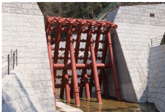
Permeable steel slit dam
